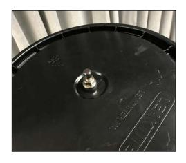
**Step 2**: Drill a ½ to ¾" hole in the center of the dirty bucket bottom to install the water filter. What size hole to drill will depend upon the type of filter is to be installed. Place the filter's mounting gasket over the filter's discharge nipple.
